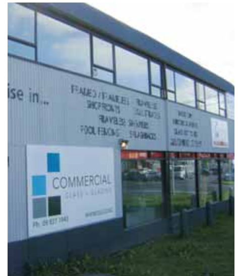
Showroom & office: Situated at 2 Crum Ave, New Lynn
